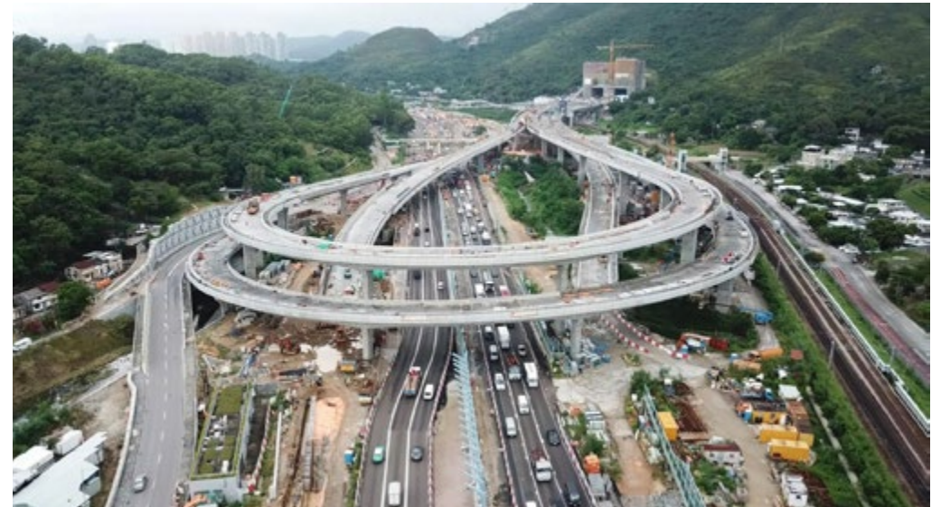
Interchange with four link roads. Meinhardt's innovative alternative designs of the viaducts provided significant savings especially in foundations.
